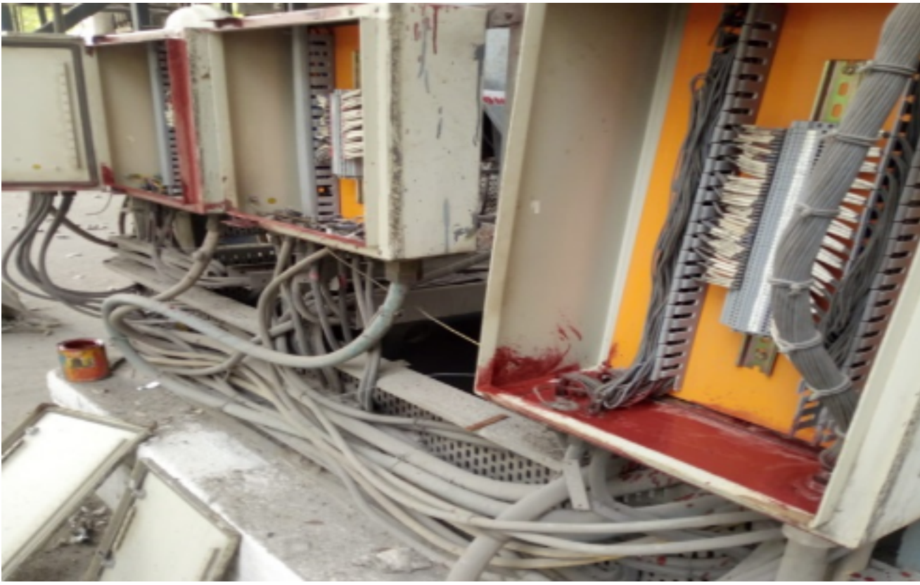
Connection Tightness Work
